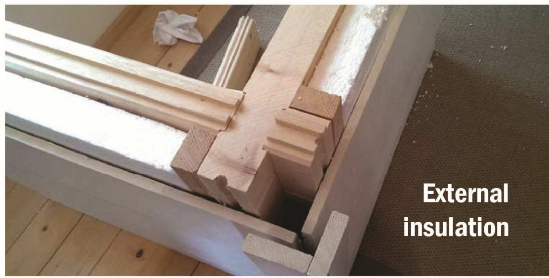
Double wall with insulation from 50 to 300mm
