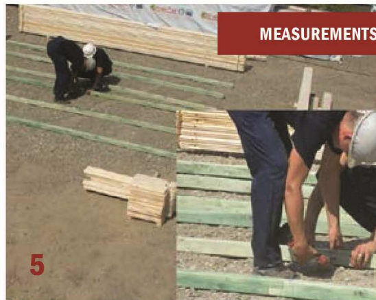
INSTALL THE LOGS
